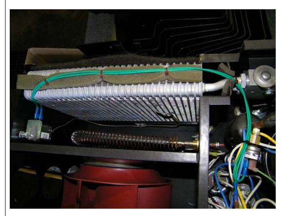
12.Re-install heat coil if it had been removed.13. Test A/C operation and return to service.
